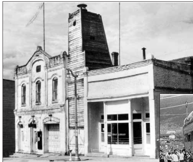
City Hall & Annex
